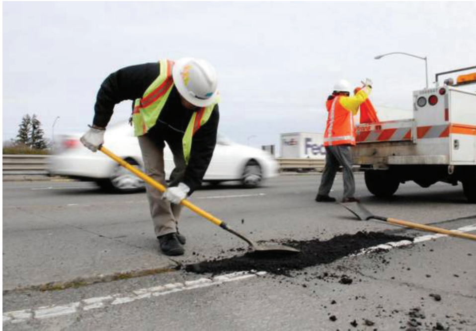
Caltrans workers fill a pothole on the Capital City Freeway. If you see a pothole developing within Sacramento County or city limits, call 311 to request a repair. Florence Low Sacramento Bee file
